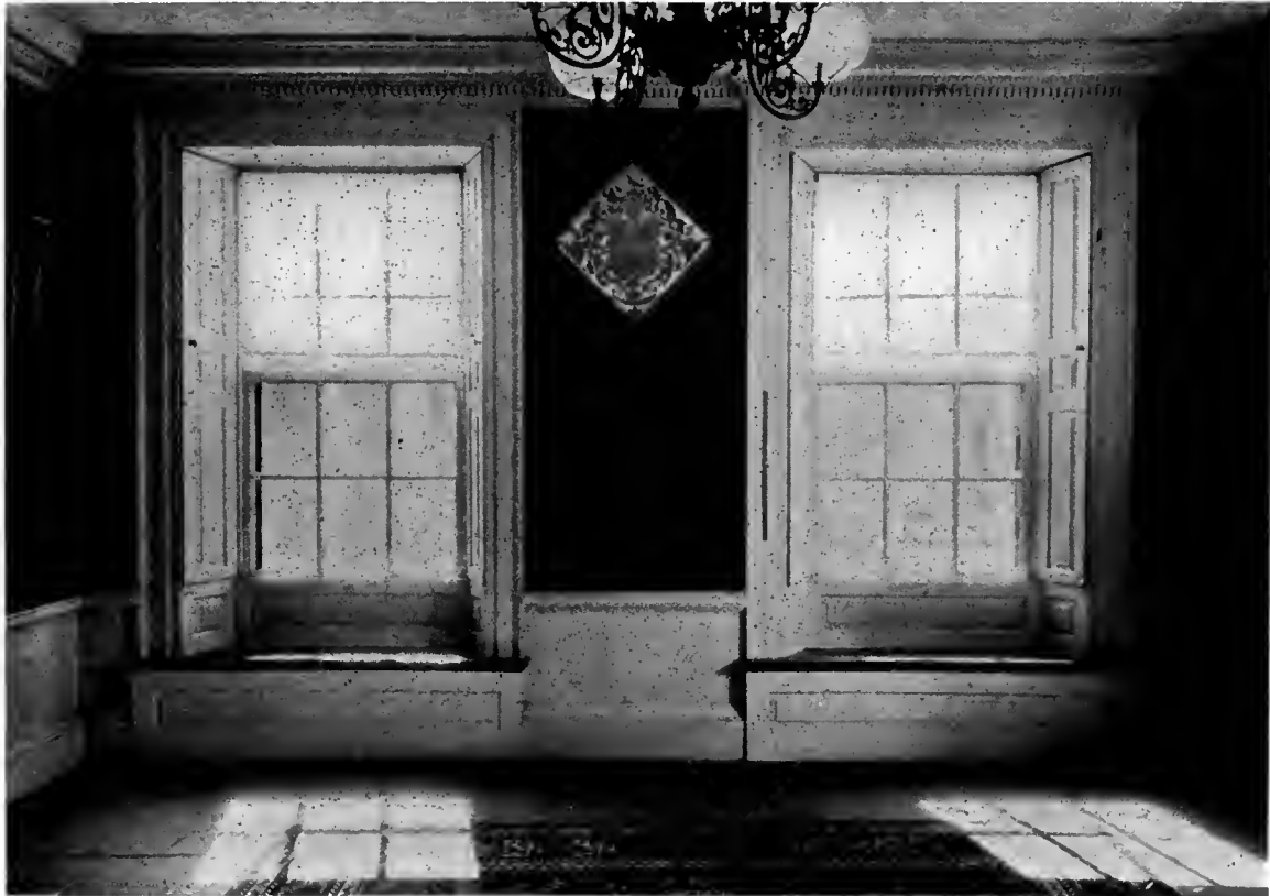
EMBRASURED WINDOWS AND SEATS, WEST PARLOR PIERCE-NICHOLS HOUSE, FEDERAL STREET, SALEM, MASS. SAMUEL McINTIRE, ARCHITECT
